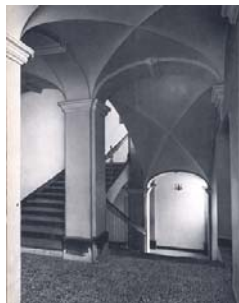
The great stairway of the seminary at Chieri as seen from the dormitory.
