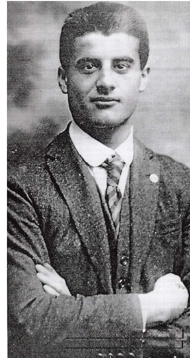
Pier Giorgio Frassati (4 July)
